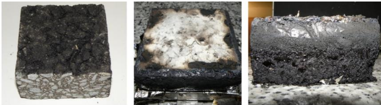
Figure 1. Pictures of asphalt pavement before and after a fire experiment from (Puente et al., 2016)
