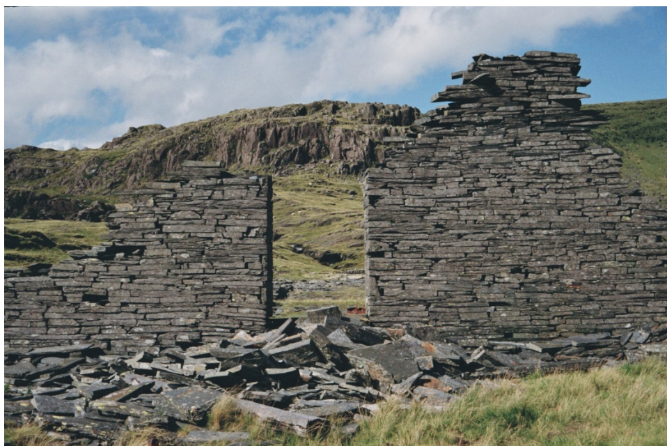
Figure 3 A doorway in the remains of the level 9 mill. Image courtesy of the author, August 2019.
