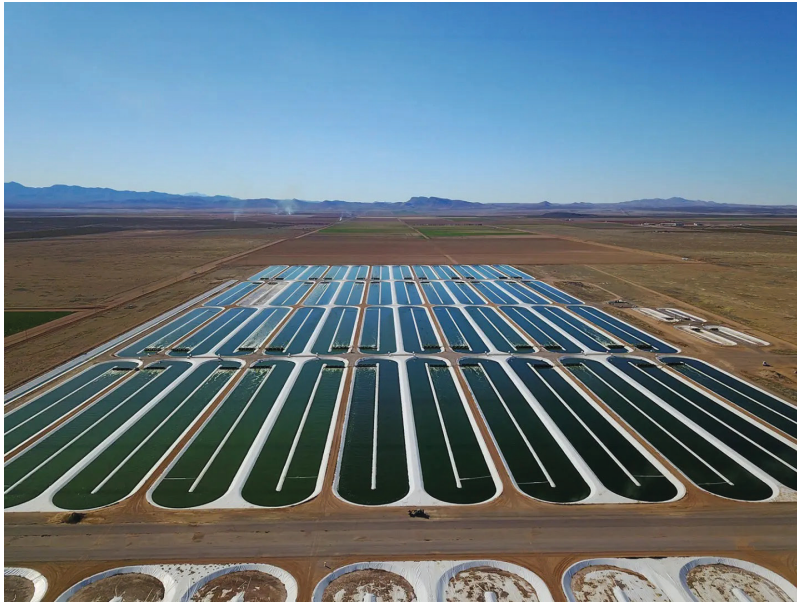
Figure 3: Some companies cultivate algae in “racetrack ponds,” large, shallow pools of microalgae that are mechanically stirred to ensure uniform sunlight and nutrient exposure. Upscaling microalgae production in areas that enjoy consistent and bright sunlight exposure could feasibly supplement or replace the petroleum supply.
