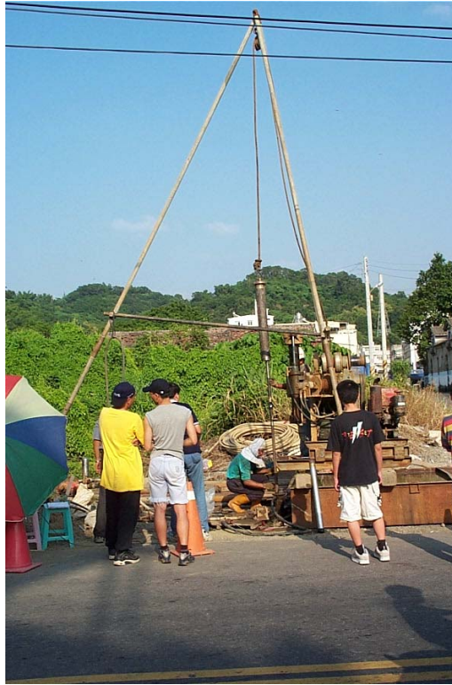
Fig. 5. Tripod supported drilled rig with a safety hammer for SPT
